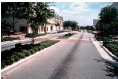
Combining a curb extension with a median shortens the crossing distance for pedestrians and create better visibility between the motorist and the person crossing. Curb extensions can alternate with on-street crossing but should not extend into the bike lane.
